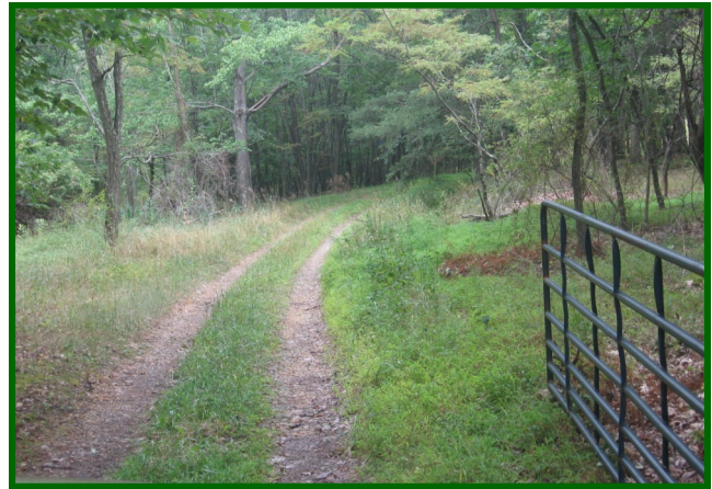
Figure 5. Properly constructed forest access road
